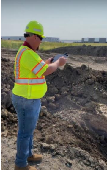
Figure 33. Utility as-built creation using Vigram viDOC
