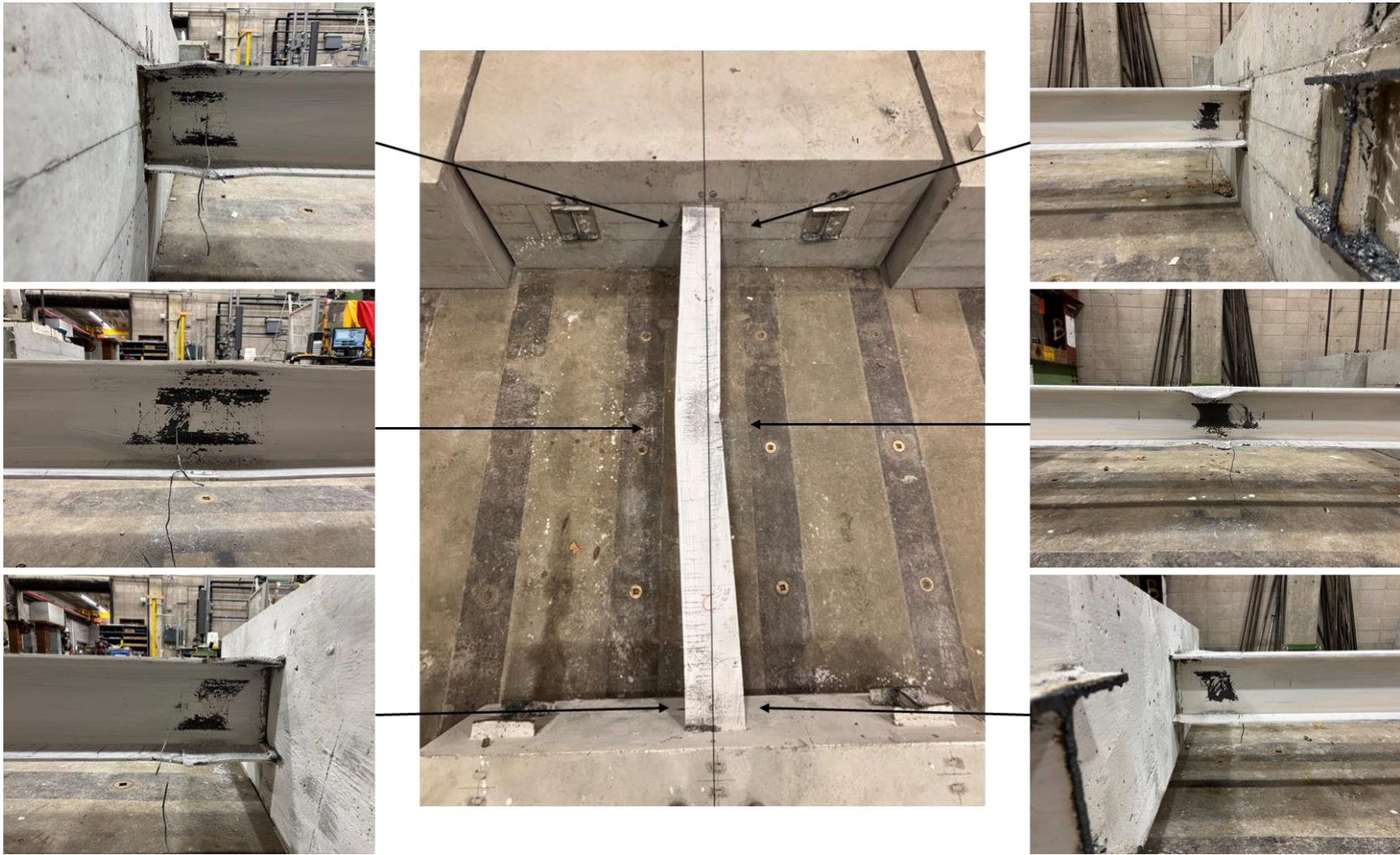
Figure 3-42. Web and flange views of pile at sections Middle, H, and Fix after testing
