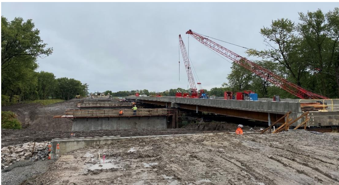
(b) Substructure of IA 1 bridge with bridge orientation
