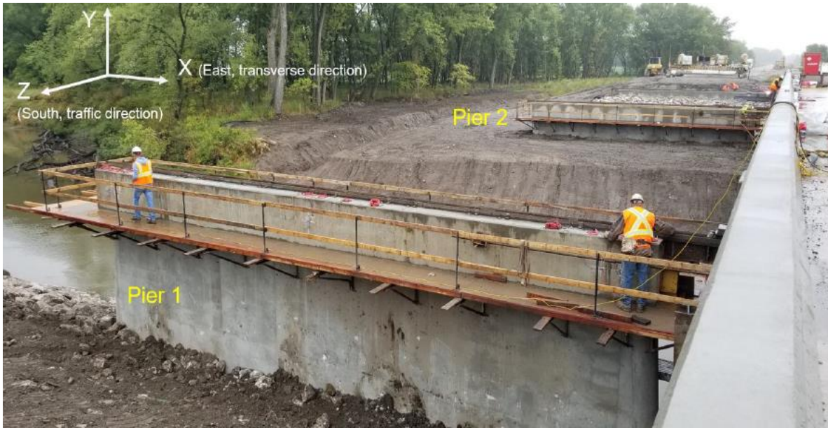
(a) Superstructure of IA 1 bridge
