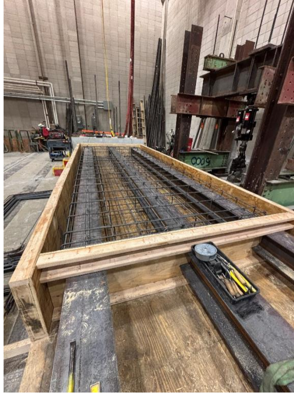
Figure 3-7. Pile encasement construction
