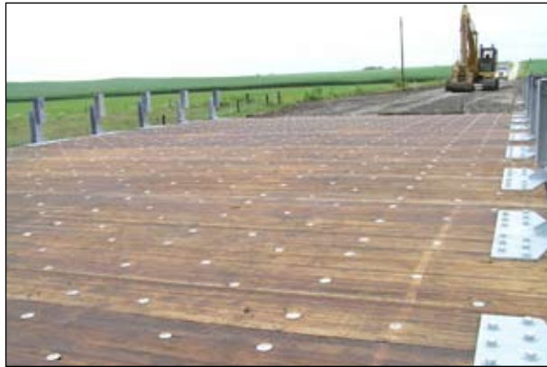
Modern timber bridge decks are typically panelized systems constructed on engineered wood products.
